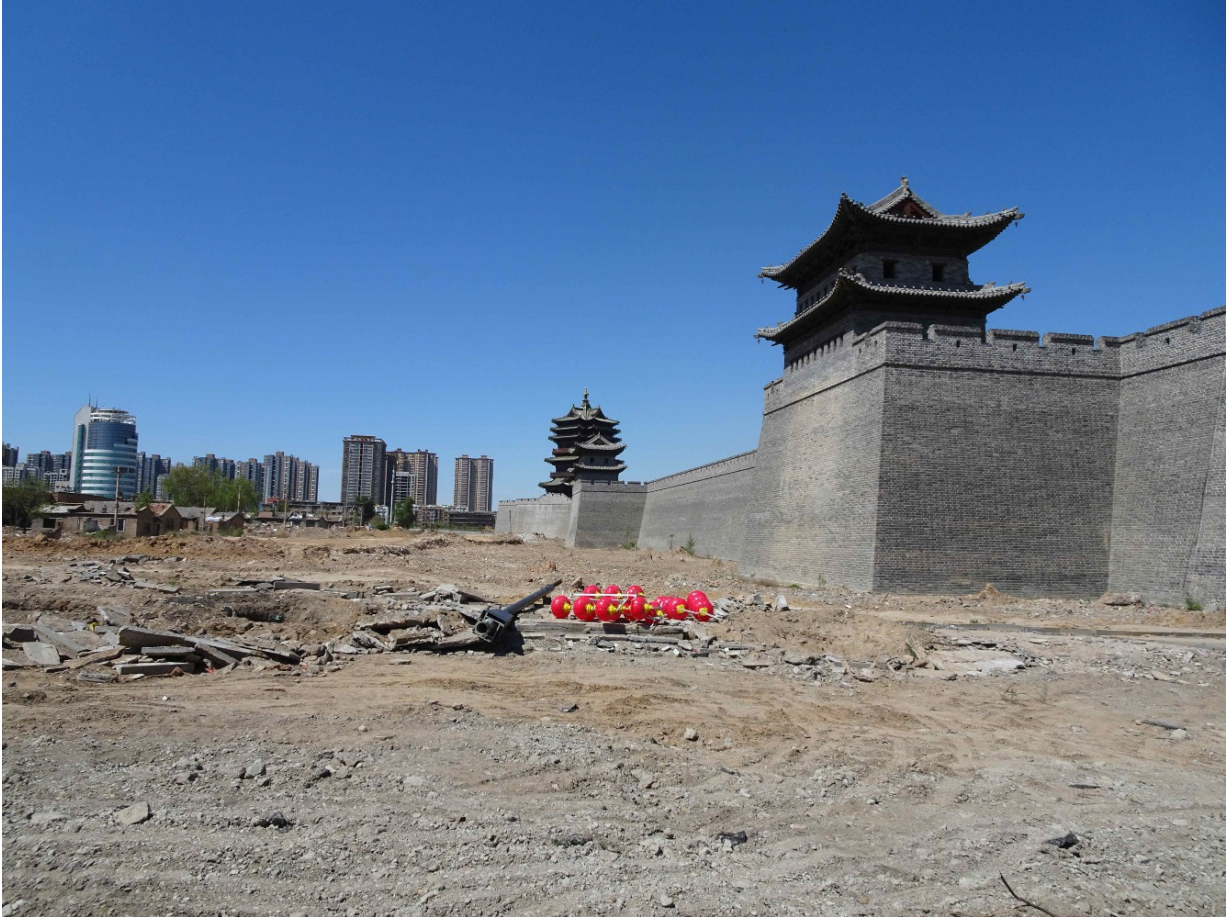
Photo 23. Construction site next to the old city wall, Datong, May 2016
