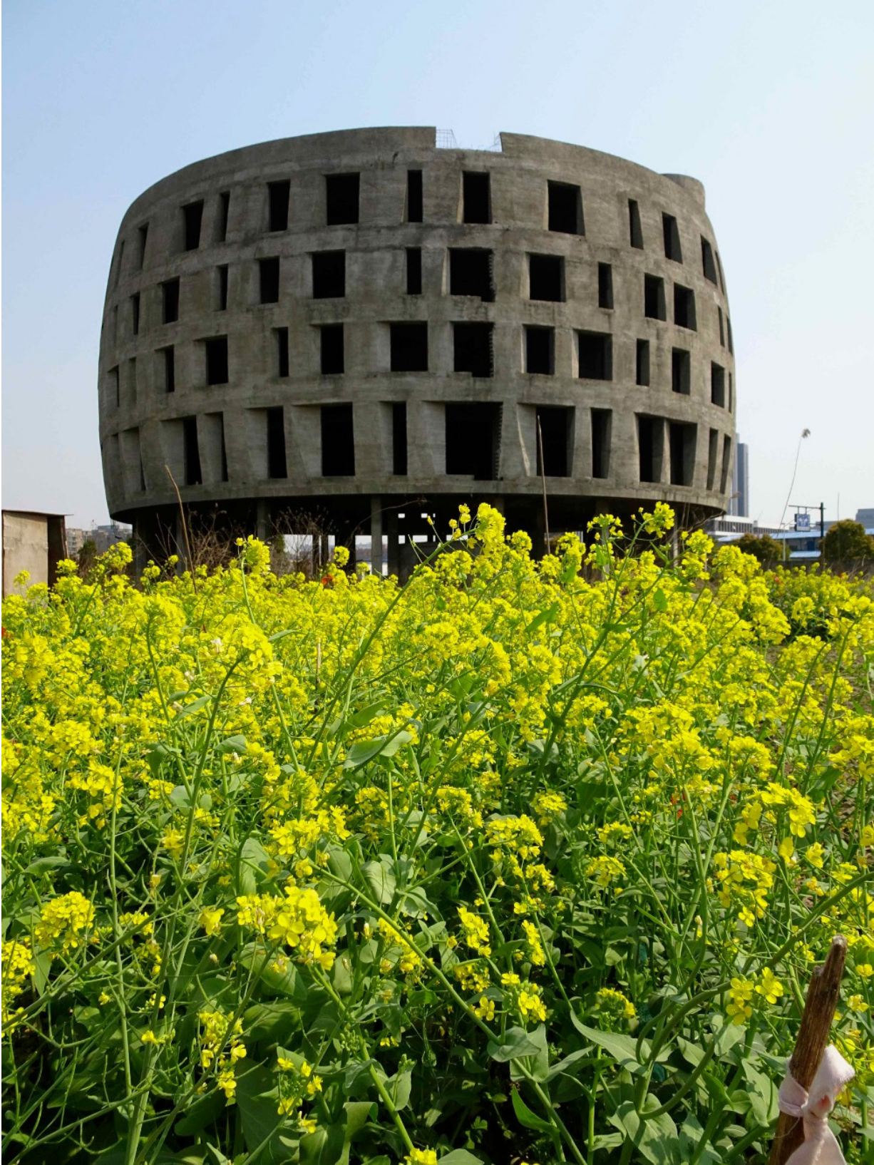
Photo 22. Abandoned unfinished building, Hangzhou, March 2016
