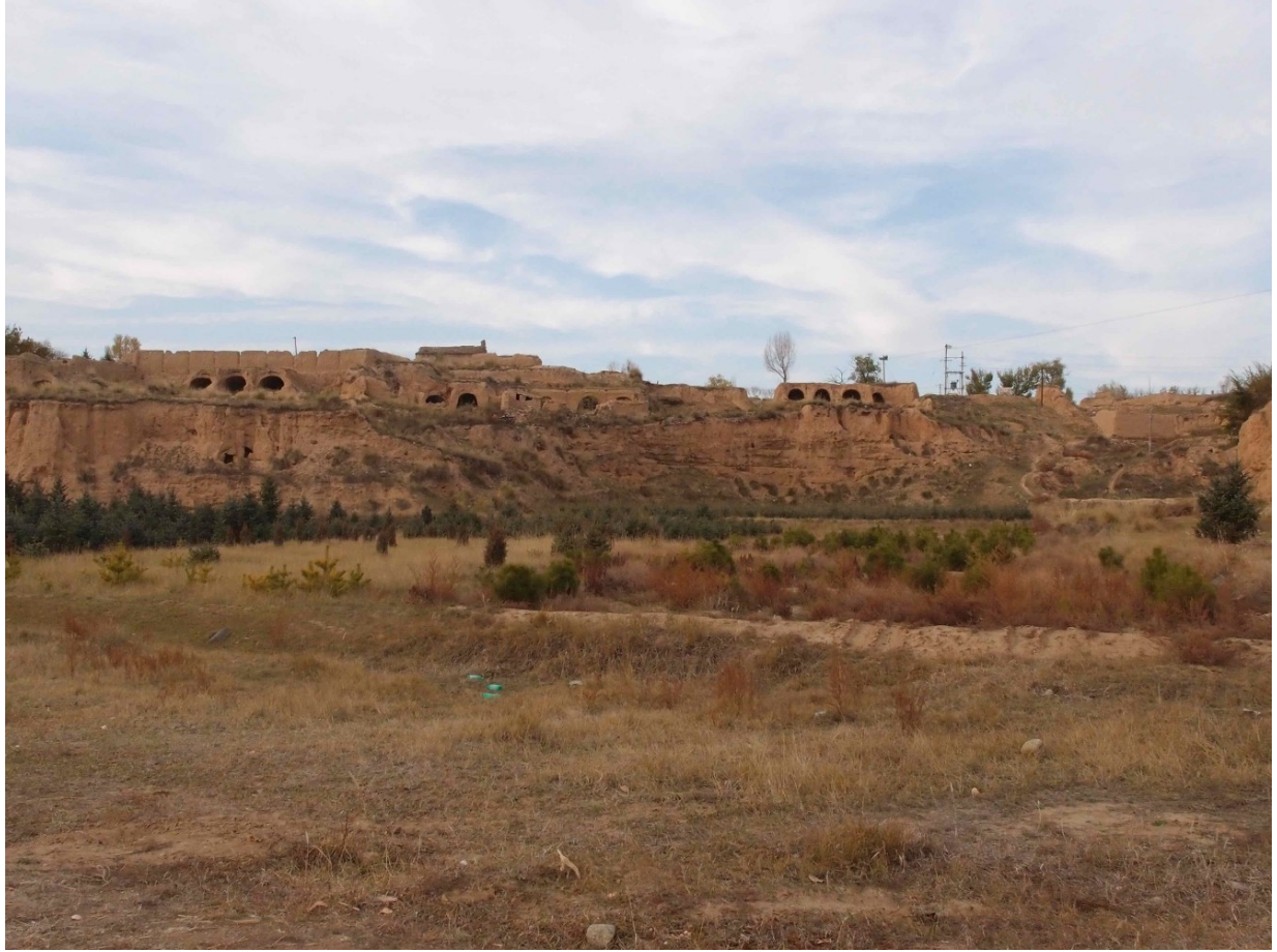
Photo 6. Abandoned villages of Shanxi province, visited in October 2015, suggest the disappearance of yaodong , troglodyte dwellings typical of the Loess Plateau of central China
