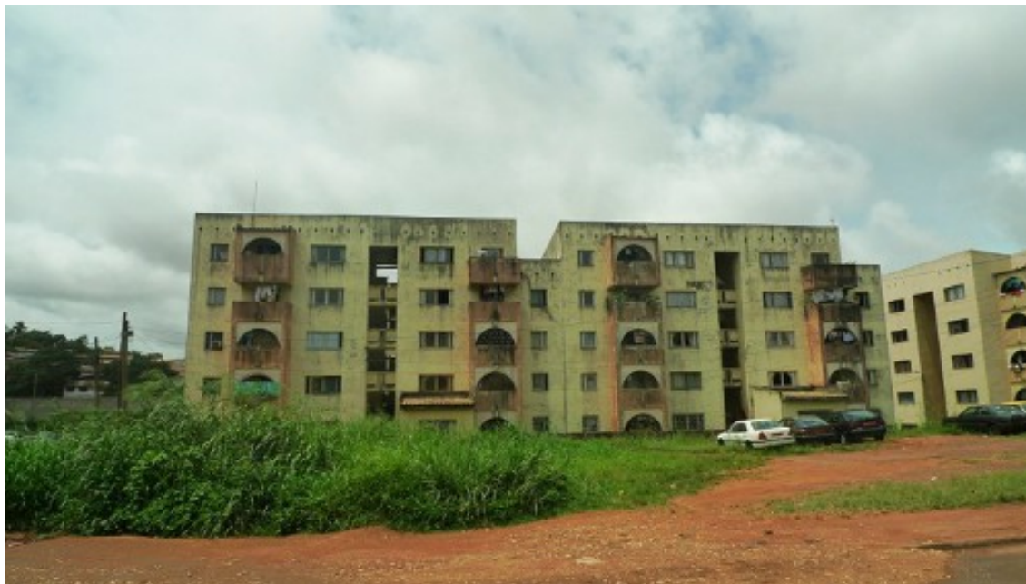
Figure 1. A collective housing complex built following independence by the Société Immobilière du Cameroun: the “Cité Verte” in Yaoundé
