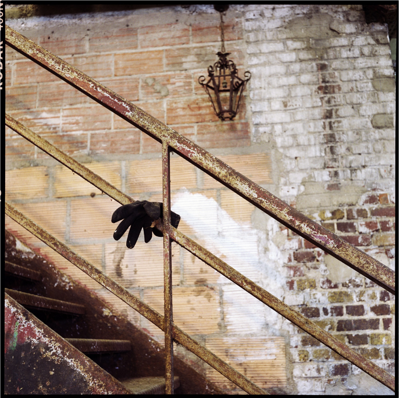
Municipal public works building, Creil.
