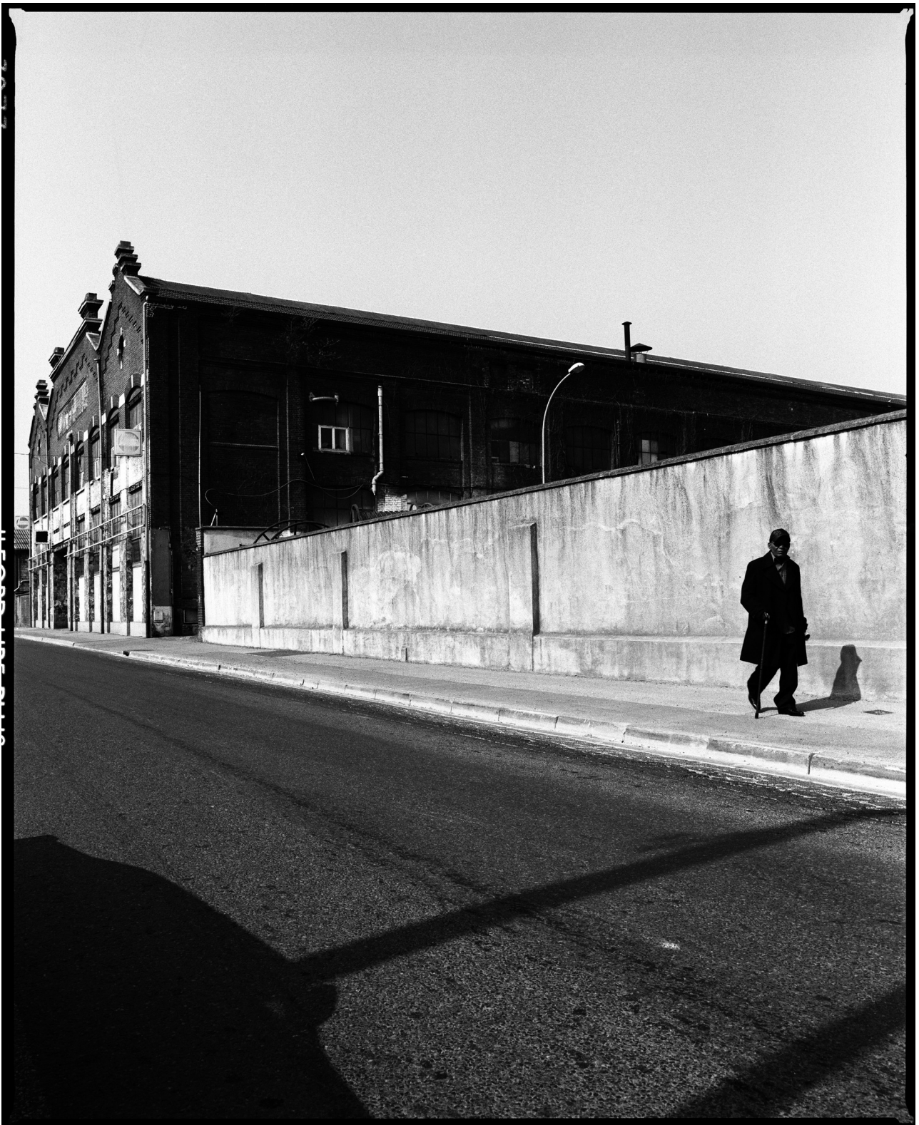
Municipal technical services, Creil. Fichet Building.
