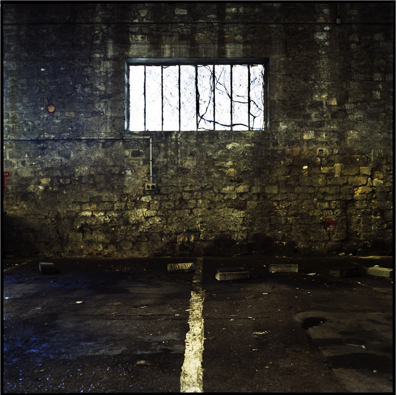
Municipal public works building, Creil.
