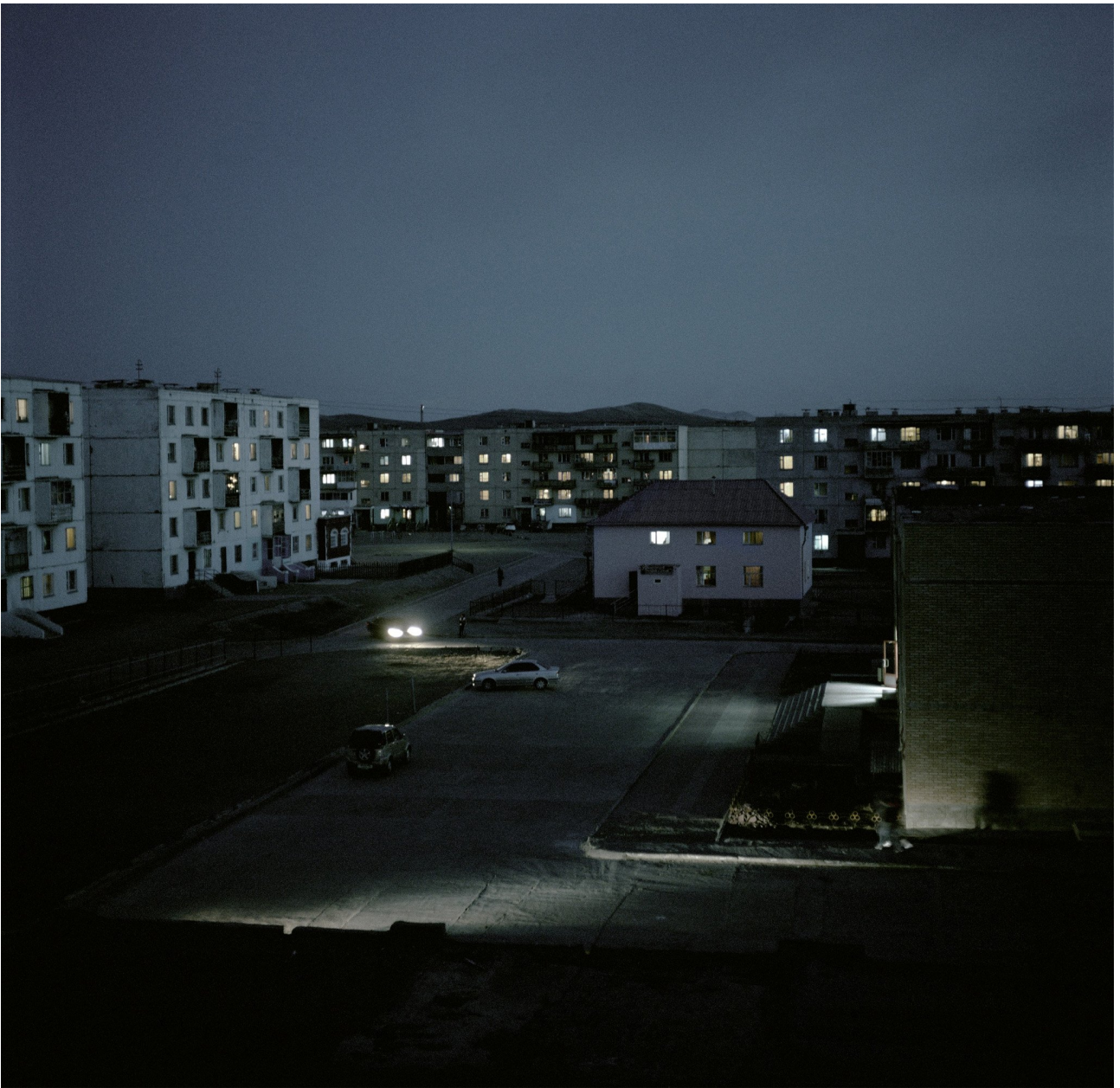
Neighbourhood of Russian-built apartment blocks.
