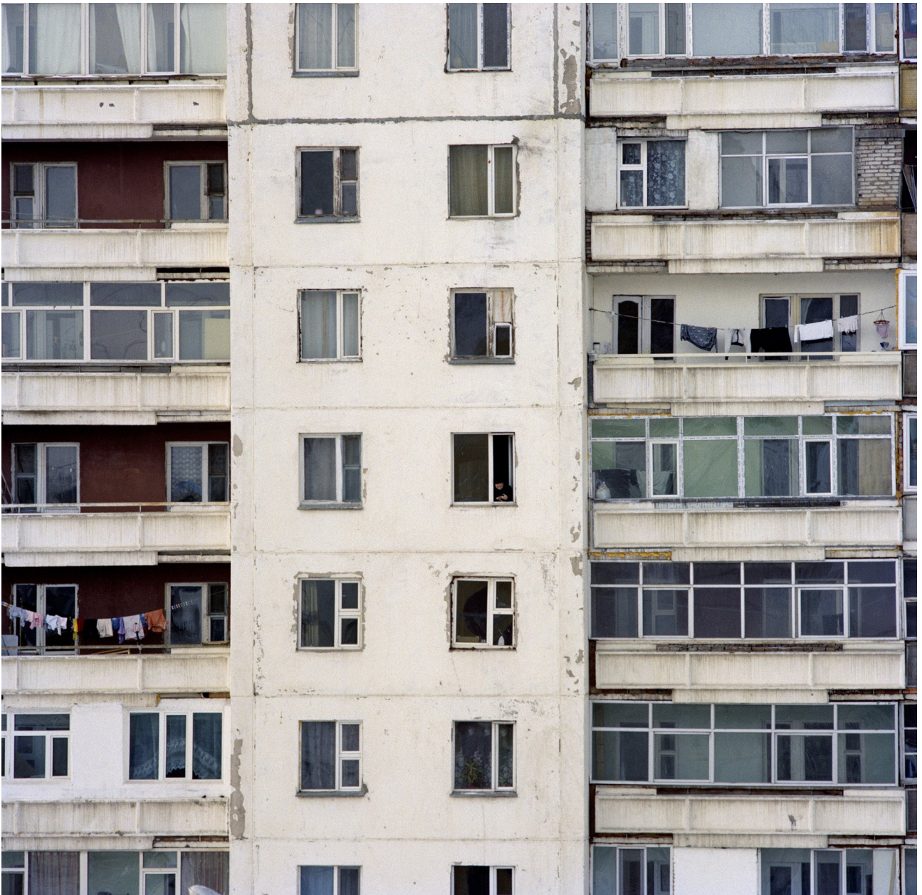
City-centre apartment block. Ulan Bator, December 2011.
